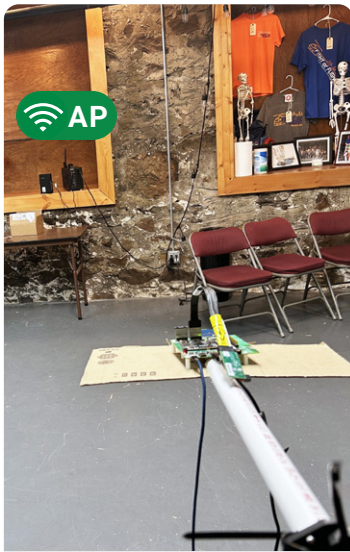
Control Room ~15 FT • Line of Sight
