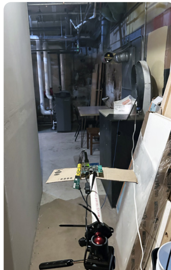
Boiler Room ~35 FT • Metal • Pumps • Elevator Shaft
